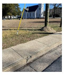
Item 2: Slab on King Carter Drive next to manhole in front of Steamboat Era Museum is shifting and cracking (New) VDOT
