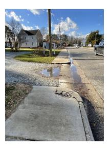
Item 5 – Start of deterioration of curb in front of Ramsey and Bugg at 4421 Irvington Road (From 2023) VDOT
