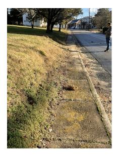
Item 11 – Sidewalk deterioration and driveway cut inconsistent with lot use at 359 Steamboat Road. (New) Town
