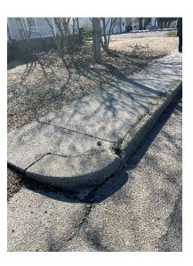
Item 6 – Deterioration of curb in several locations between gas station at 4525 Irvington Road and the Post Office (From 2023) VDOT
